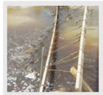
Custom curtain method used to capture colloidal clays and organic muck
