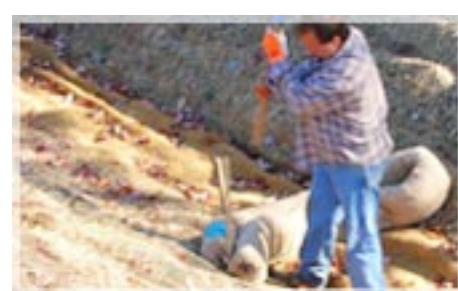
Installation of jute netting and erosion control blankets in swale
