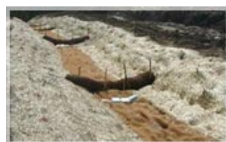
Contaminated storm water flows into swale; clean, crystal clear water flows out into wetland
