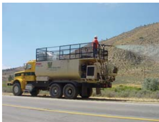
Photo: Selby's Soil Erosion Control Co.
