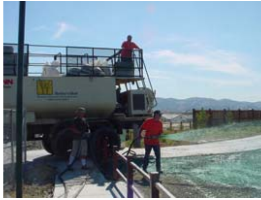
Photo: Selby's Soil Erosion Control Co.
