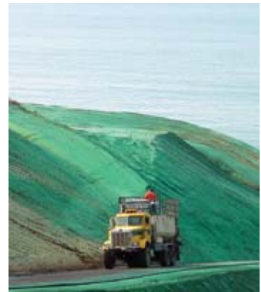
Photo: Selby's Soil Erosion Control Co.
