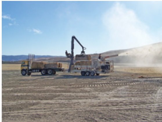
Photo: Selby's Soil Erosion Control
