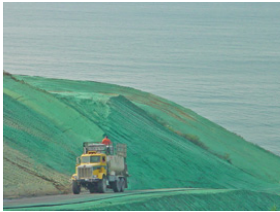
Photo: Selby's Soil Erosion Control
