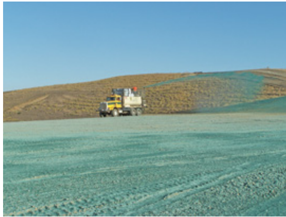
Photo: Selby's Soil Erosion Control
