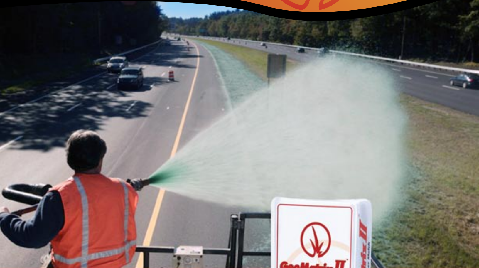
GeoMatrix II being applied from tower
